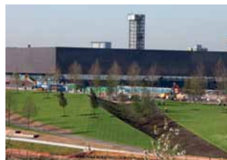
The Park's new energy infrastructure will reduce carbon emissions
